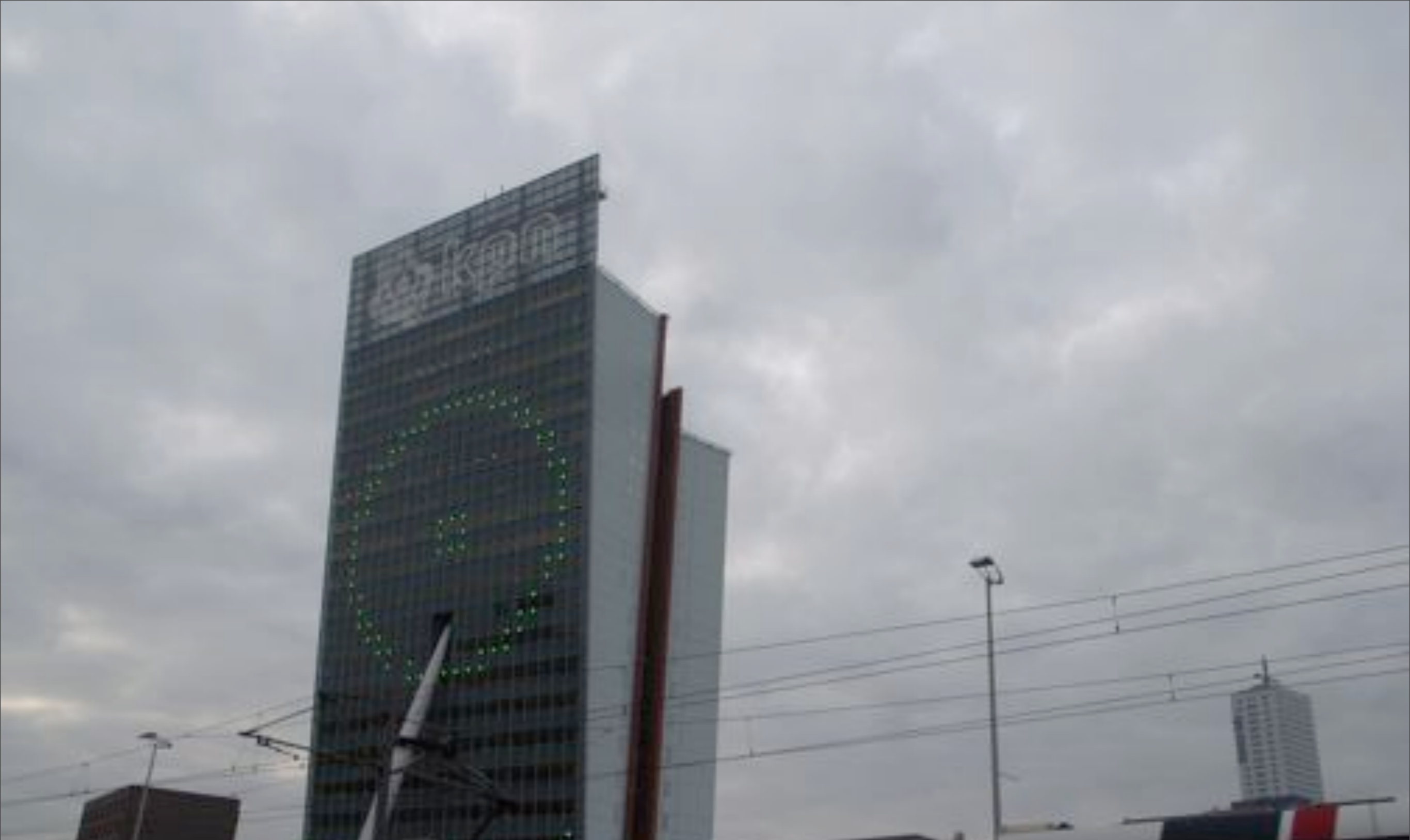
Interactive facade (KPN building, Rotterdam)
